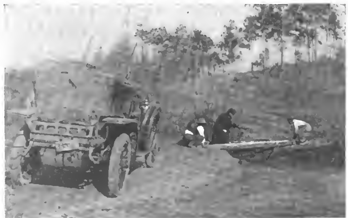
BUILDING A TRESTLE OVER A PATCH OF QUICKSAND;
